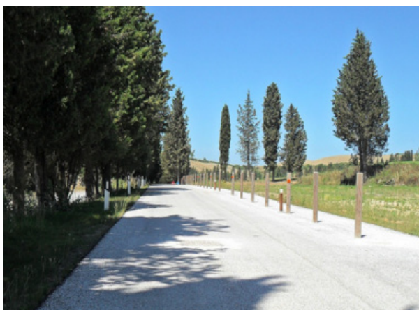
Trattamento Natural Pavement
